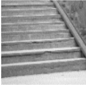
A wheeling channel makes it much easier to get from street level to the front door
